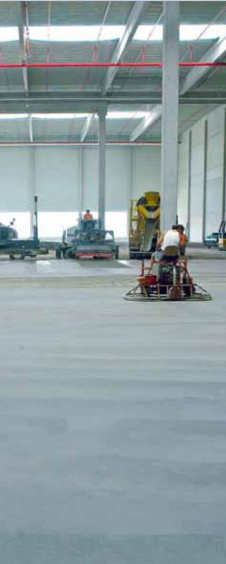
To recognise an unintended air pore content in concrete which could have a negative effect when the surface is smoothed, random testing of air pore content is advisable. Air pore contents below 3.5 % are deemed uncritical.
